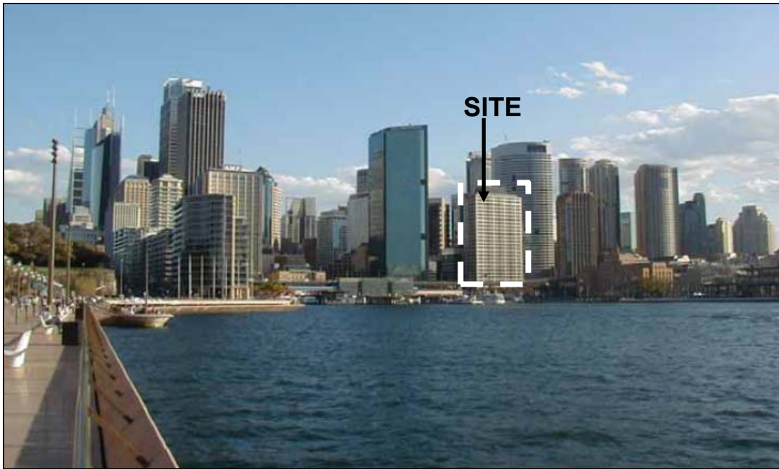
Figure 2 – The existing development on site as viewed from the East Circular Quay forecourt
