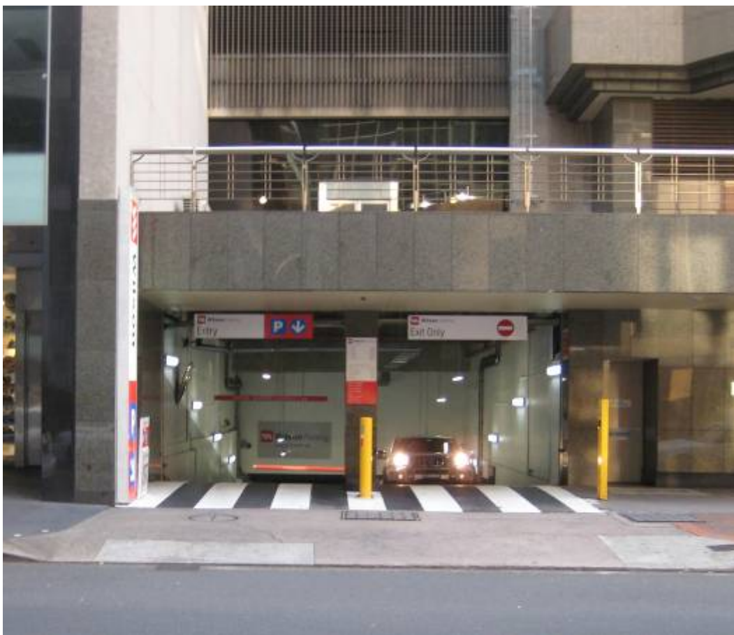
Figure 8 – The existing vehicular egress/ingress to the site from Pitt Street
